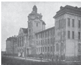
Picture 1: The building of the only eight-grade upper “real” school in Southern Transdanubia, the State Upper “Real” School in Pécs (1915) (Source: Gallovich 1915)
